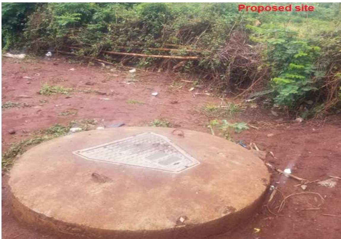
Plate 12: Manhole adjacent to the proposed site
