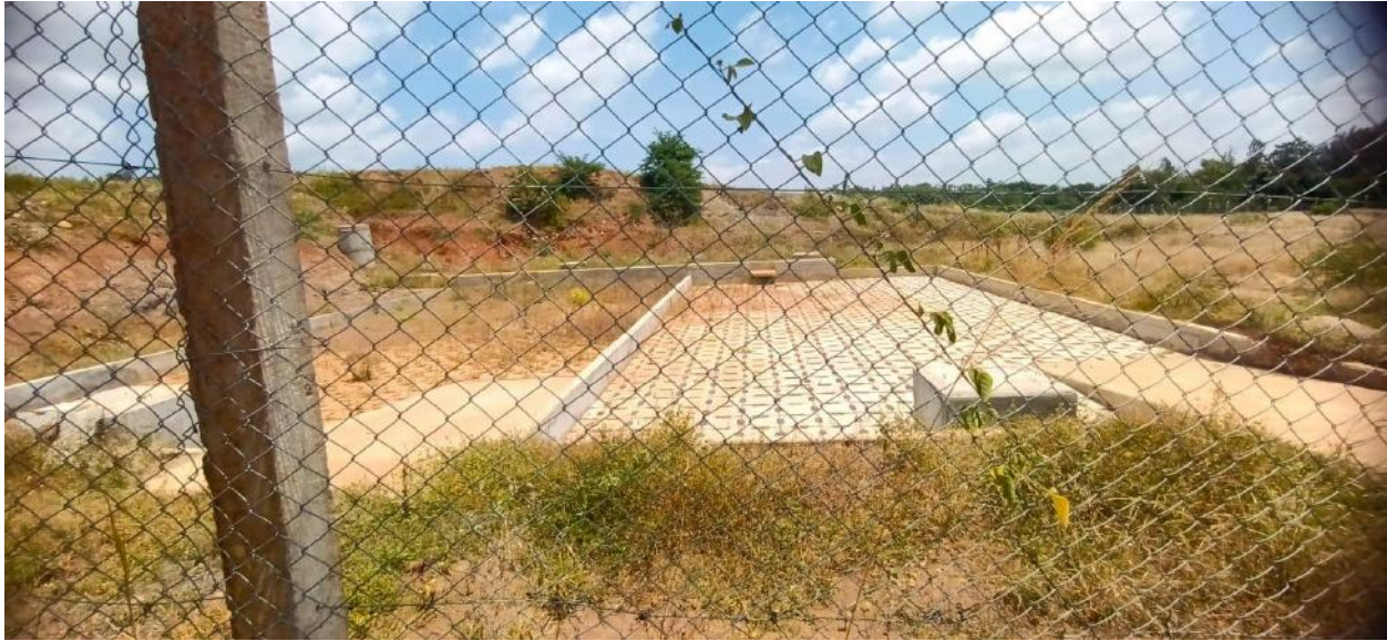
Figure 4: sewer adjacent to the proposed solid waste management site
