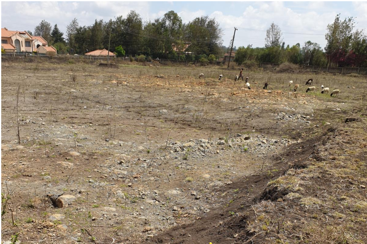
Plate 1 Excavated section of the proposed project site
