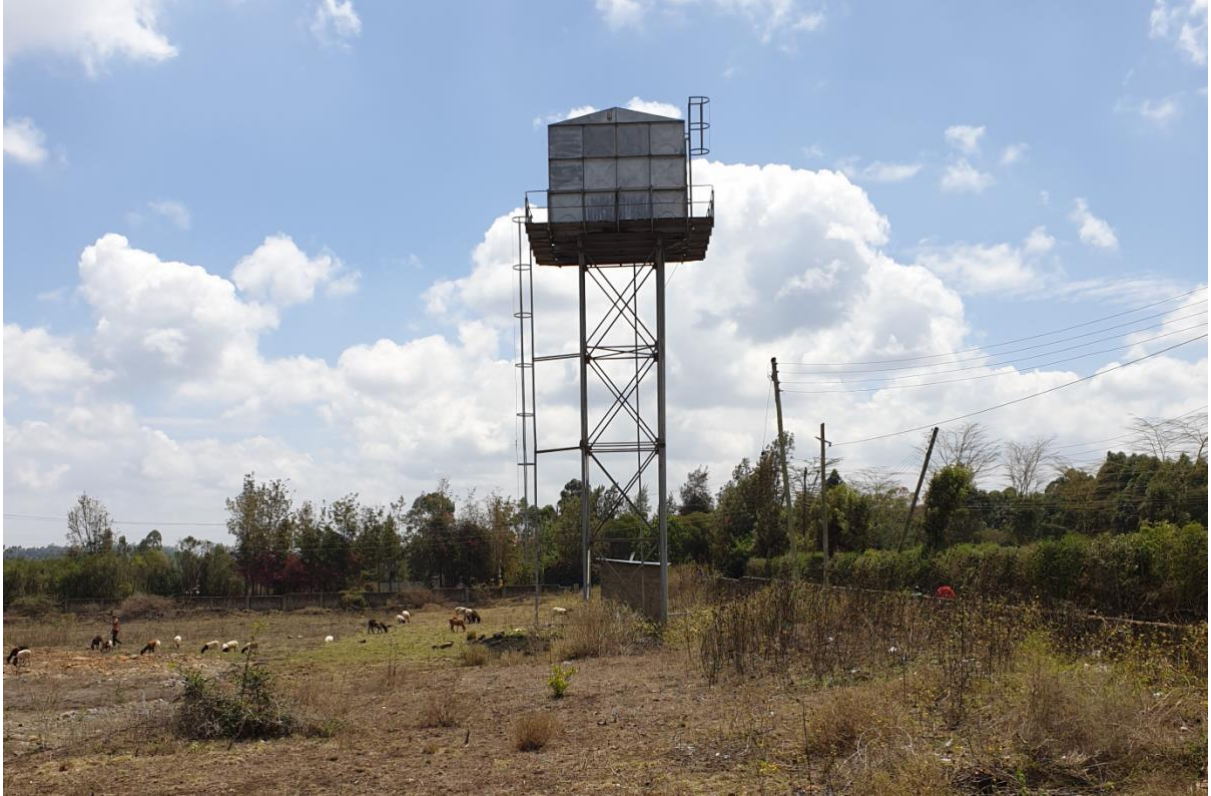
Plate 2 Existing borehole and water tank on the proposed project site
