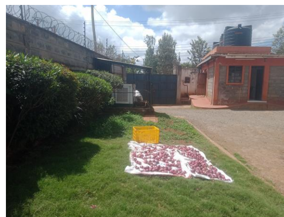
Plate 1(d): Part of the existing building.
