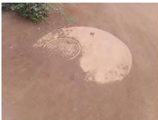
Plate 9: Sewer line manhole at the entrance to the proposed site.
