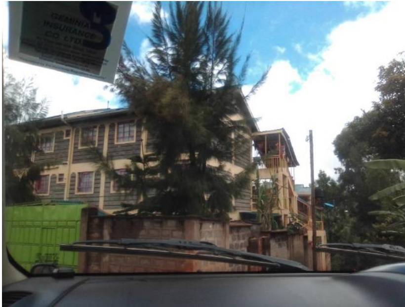
Figure 3-5: Multiple Storey Building in the project area
