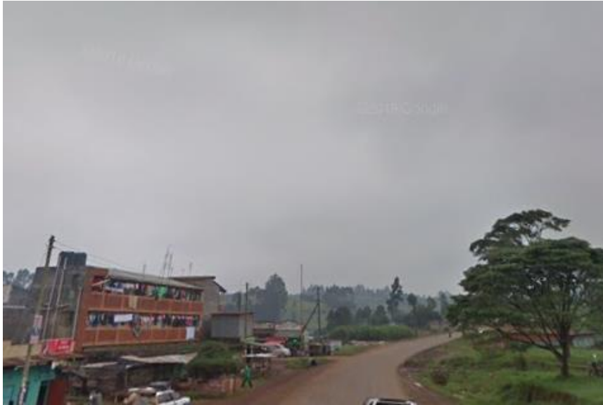
Figure 3-3: Road to the proposed project site Kangari-Kaharati Road
