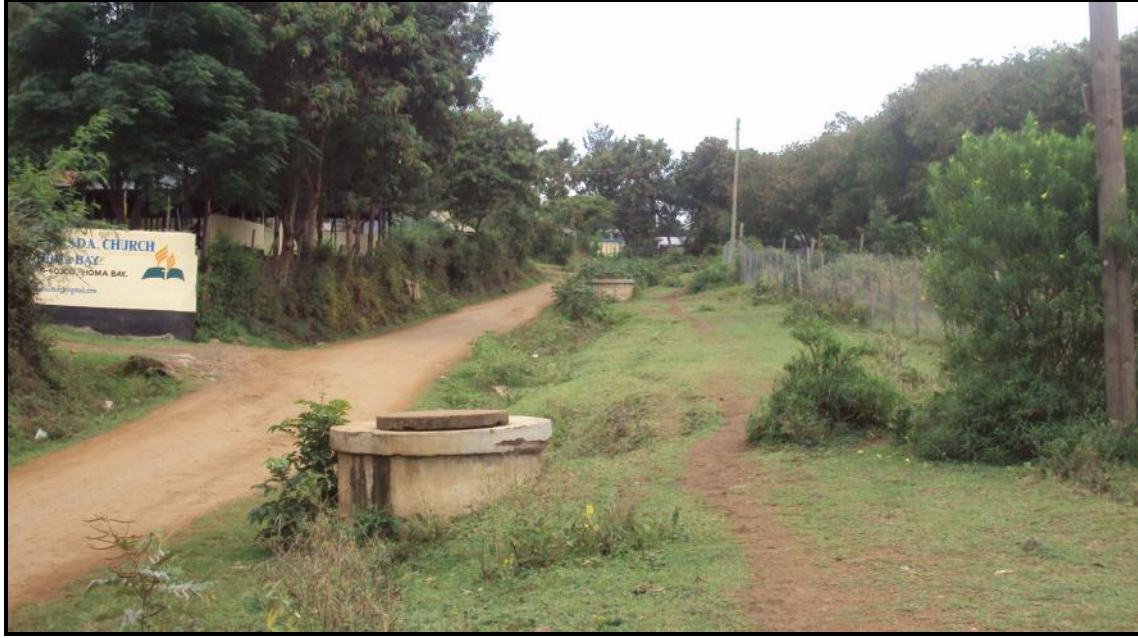
Figure 13: Main sewer trunk line adjacent to the proposed project site.
