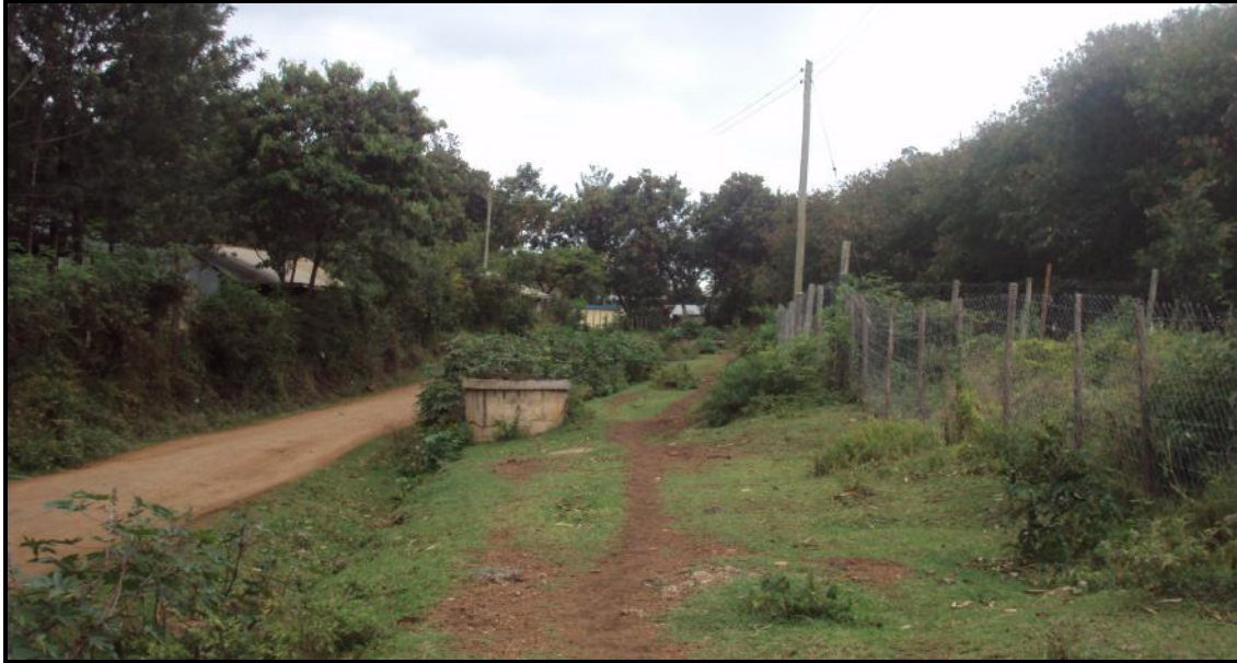
Figure 11: KPC power line within the vicinity of the propose project site.
