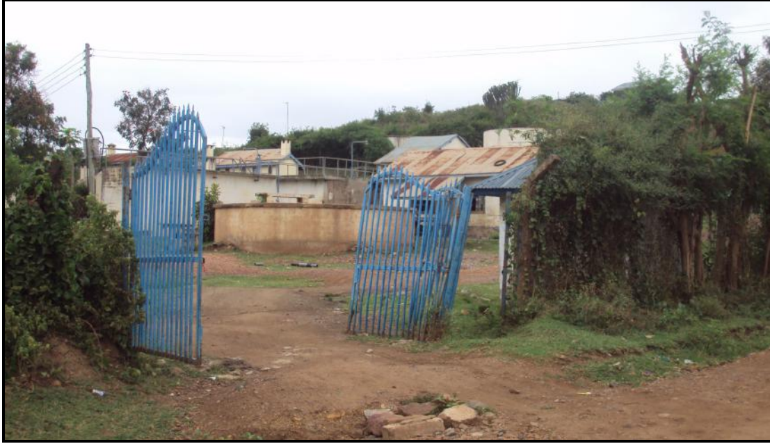
Figure 12: HOMA WASCOWater treatment plant next to the proposed project site.
