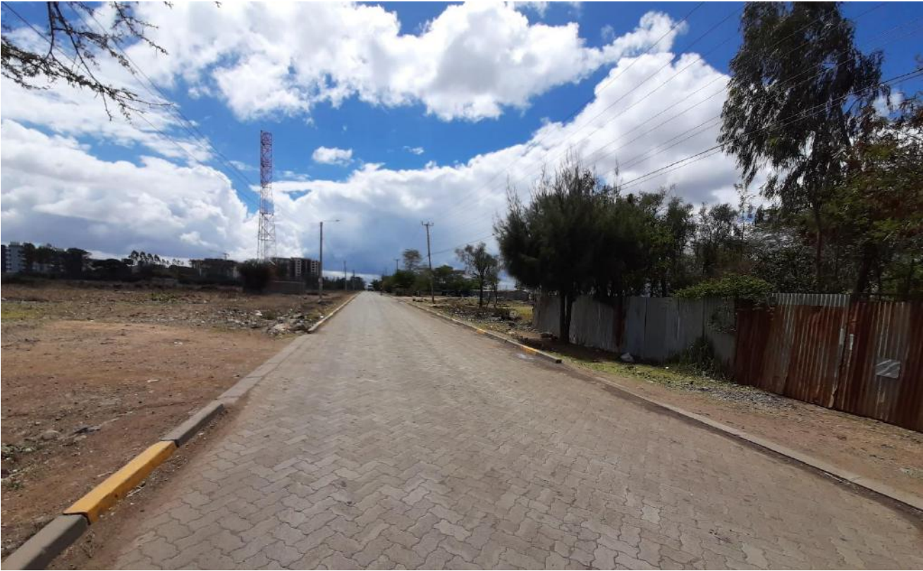
Figure 3: Access road to the proposed project area
