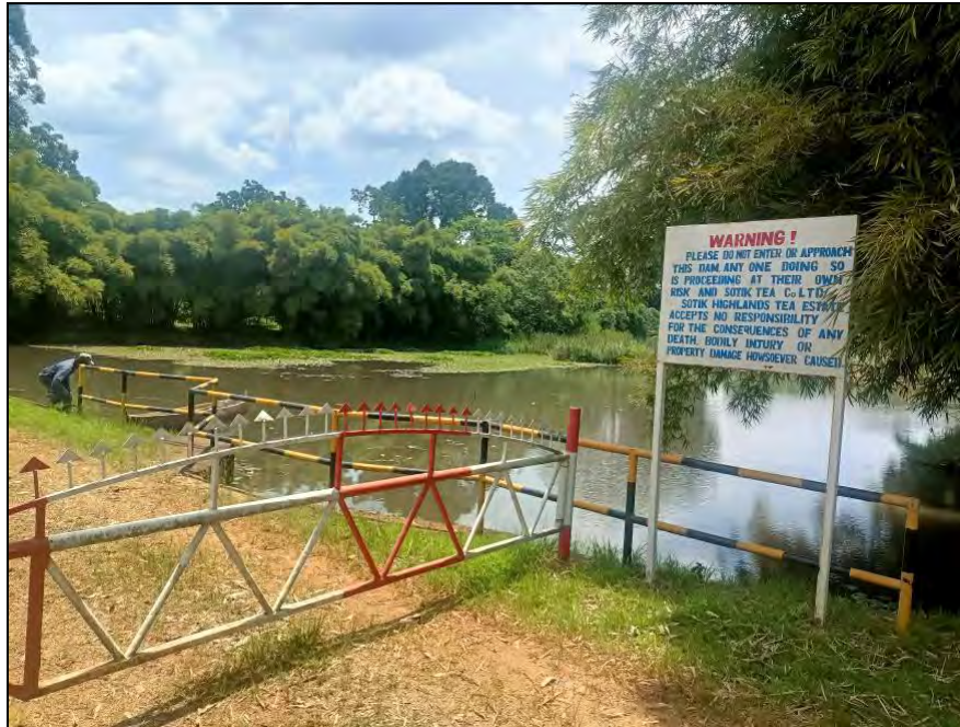
Figure 8-2: A barrier and warning sign to limit access at Kapkoya dam. (Note the vegetation cover maintained around the impoundment)
