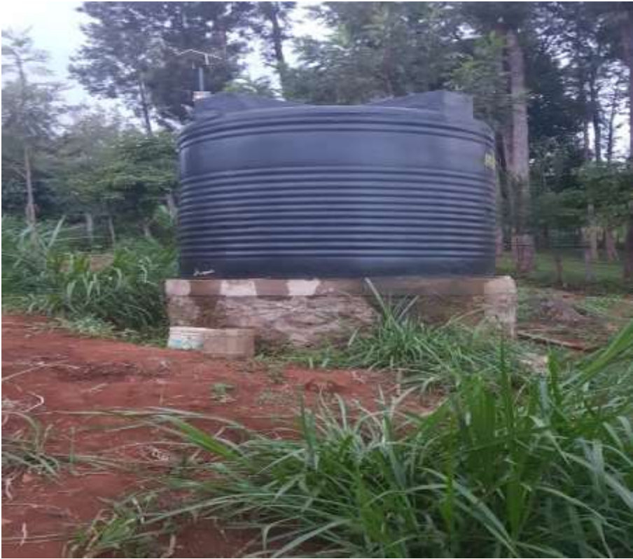
Figure showing one of water storage tanks
