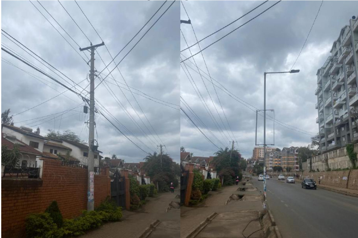
Plate 4. 4: Power lines and Street lights along the access road
