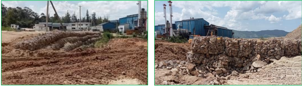
Figure 10: Gabions constructed within the proposed project site to prevent soil erosion (Source: site visits, July 2022).
