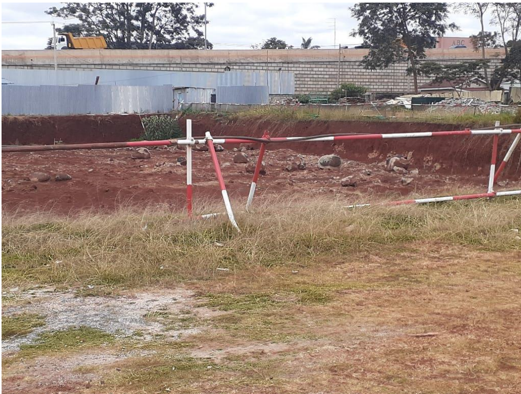
Plate 2: Construction status at the site – showing excavations
