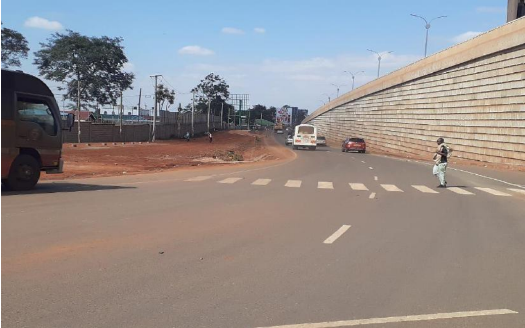
Plate 7: Waiyaki Way and the Express Way (Project site to the left)
