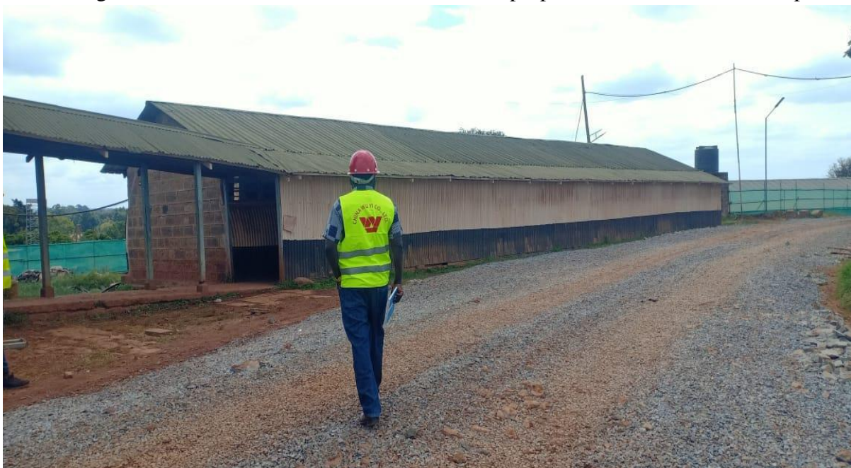
Plate 1: Part of the remaining Building to be demolished
