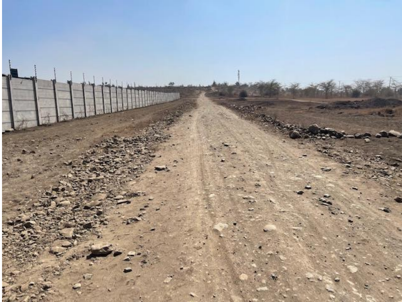
Photo 5: Road currently serving the project site
