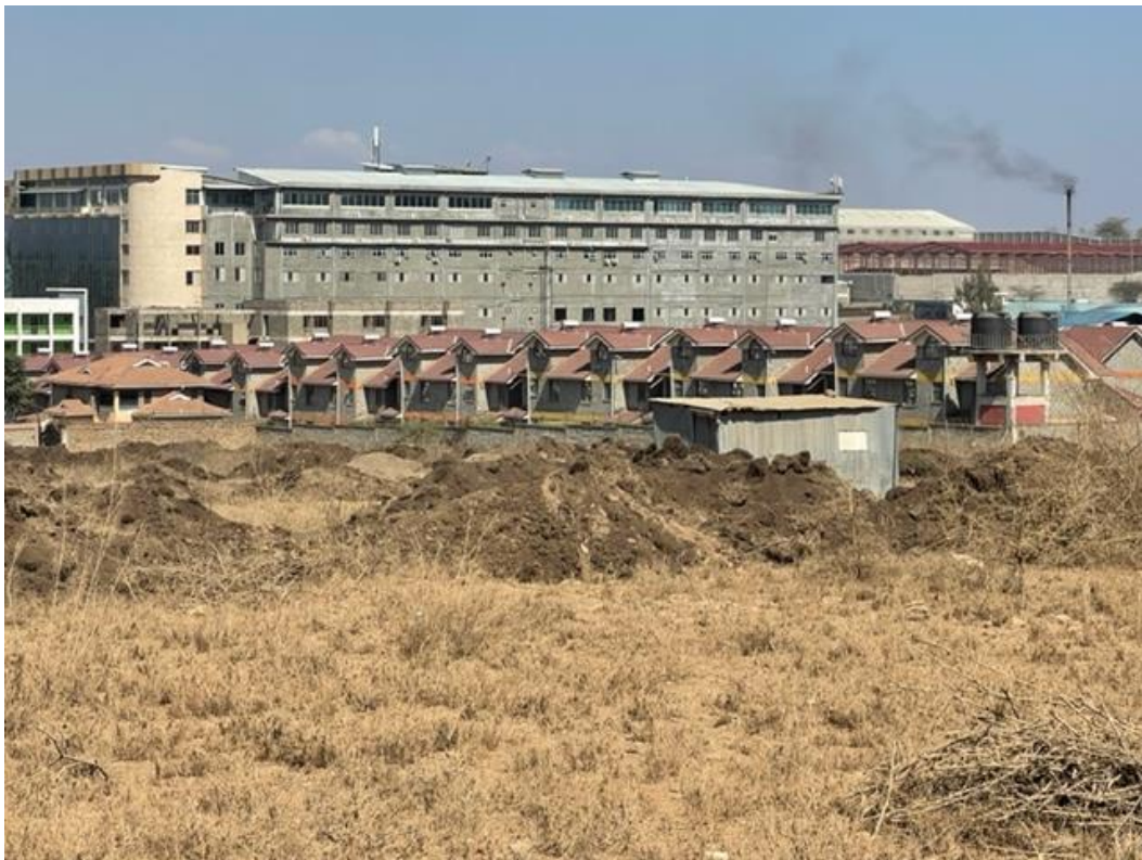
Photo 3 & 4: The similar neighbouring developments undergoing construction
