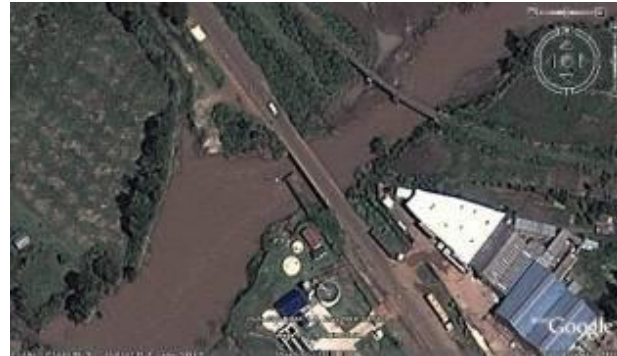
Nzoia River crossing at Mois Bridge
