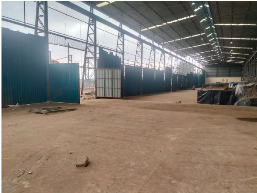
Figure 2: Existing godown within which mill will be installed
