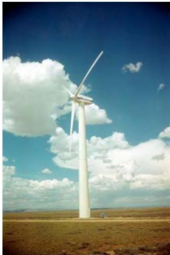
Figure 10: Wind turbine. Source: DOE/NREL ( http://www.nrel.gov/data/pix )
