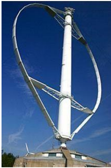
Figure 13: A typical Darrieus Turbine (Source: www.windpowerengineering.com )
