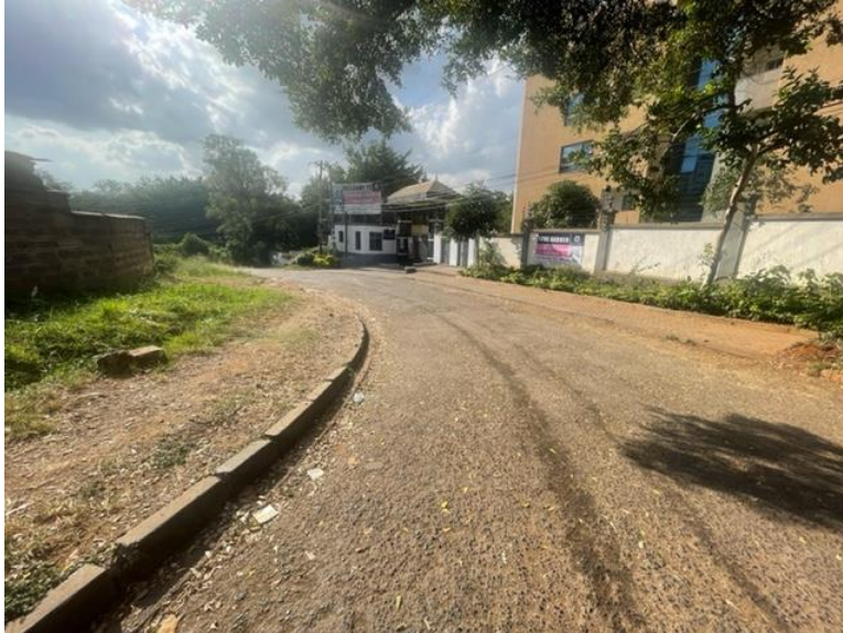
Photo 6: A section of Gatundu Crescent currently serving the project site
