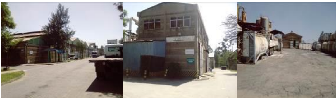
Figure 2: Existing site conditions at OPAL
