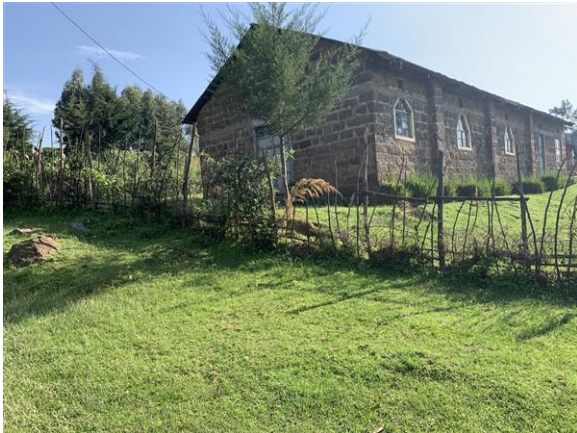
Plate 5-4: PEFA Sachangwan church located close to the project site (810132.46E; 9977160.87S)
