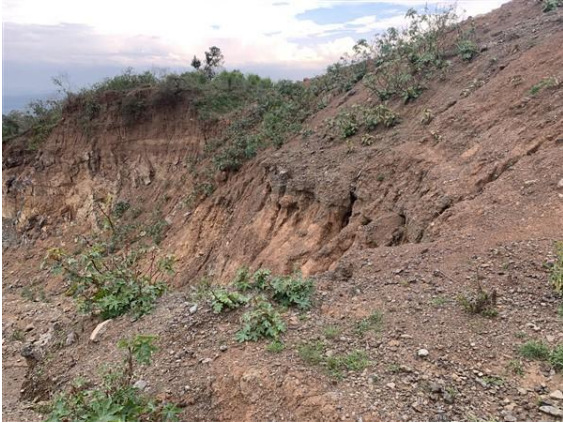
Plate 5-1: Section of the site showing rill erosion
