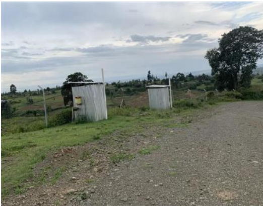
Plate 5-8: Pit latrines on site for managing fecal waste
