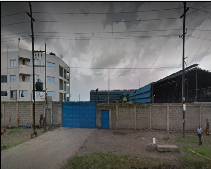
Endmore Steel Millers Factory in syokimau Mavoko Subcounty
