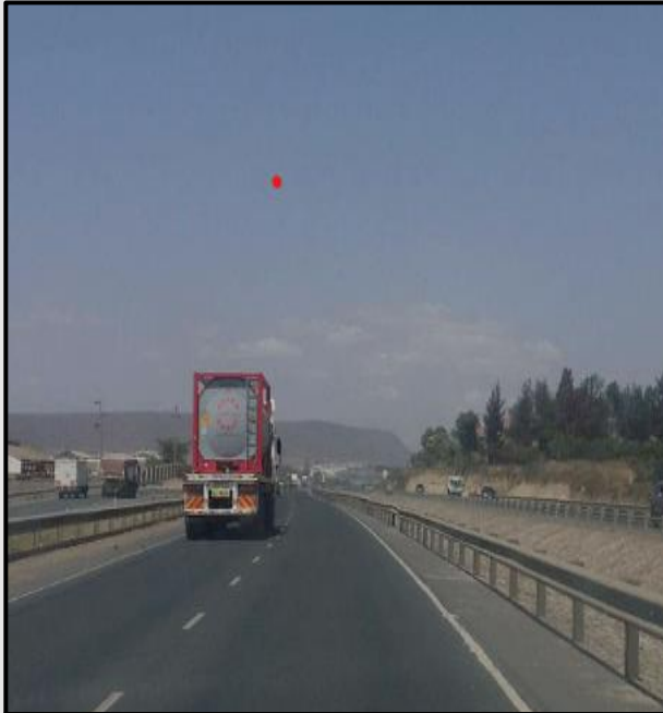
Section of Mombasa Road at the Namanga interchange
