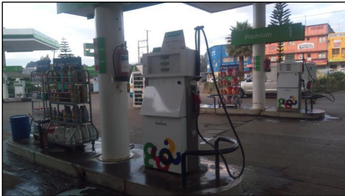
PLATE 9: canopy and pumps to be removed
