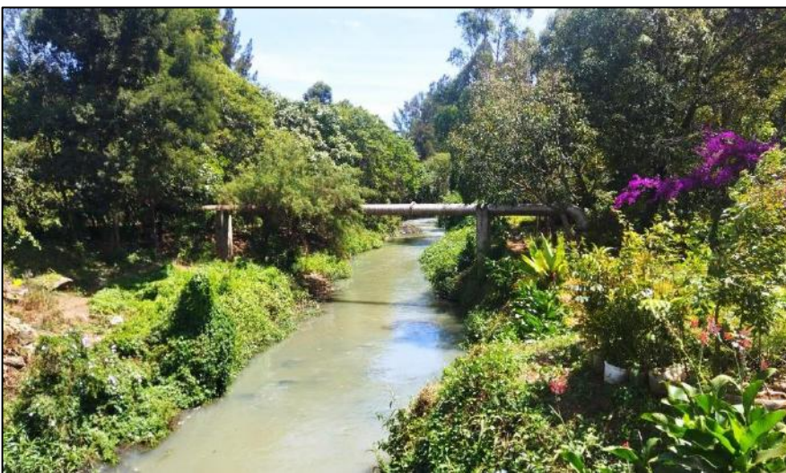
PLATE 8: a public sewer line passing across River Sossiani 400 meters from proposed site
