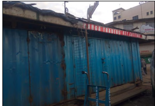
PLATE 10: a Jua Kali shade to be demolished
