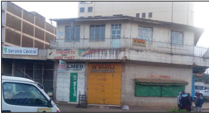
PLATE 11: one storey building to be demolished
