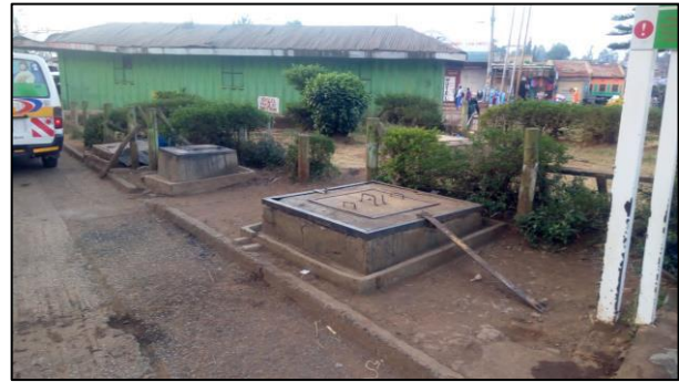
PLATE 12: underground storage tanks covers to be removed
