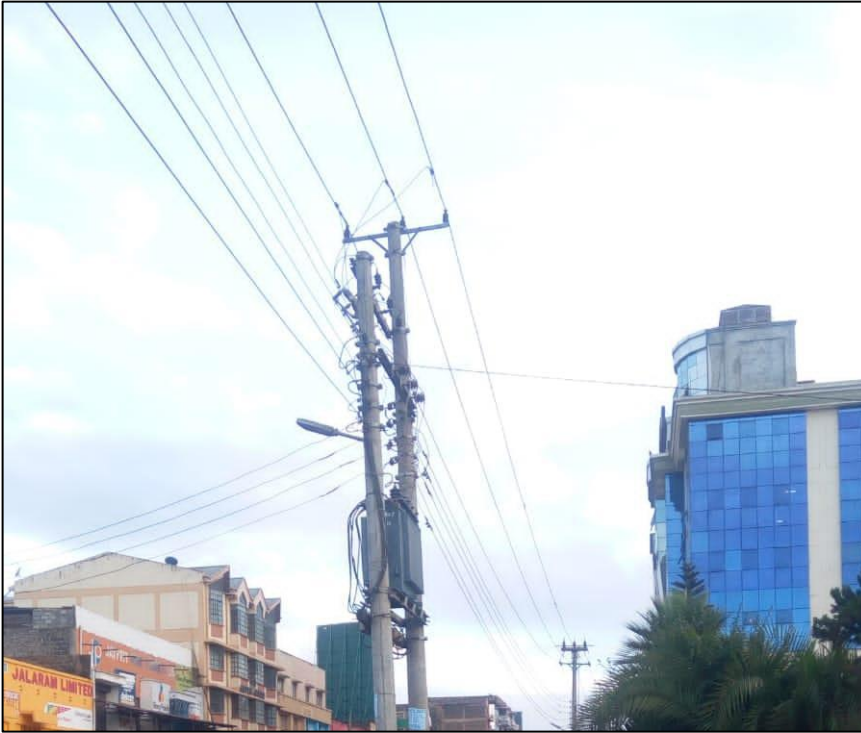
PLATE 16: electricity power line passing along Ronald Ngala Street
