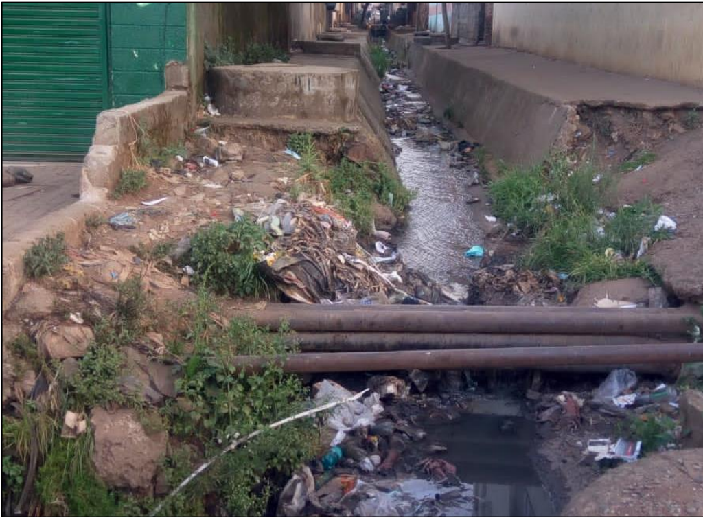
PLATE 17: water pipeline serving around the proposed site
