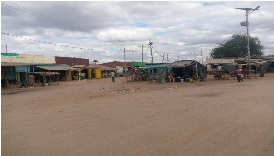
Plate 9 Power lines at Kavisuni town
