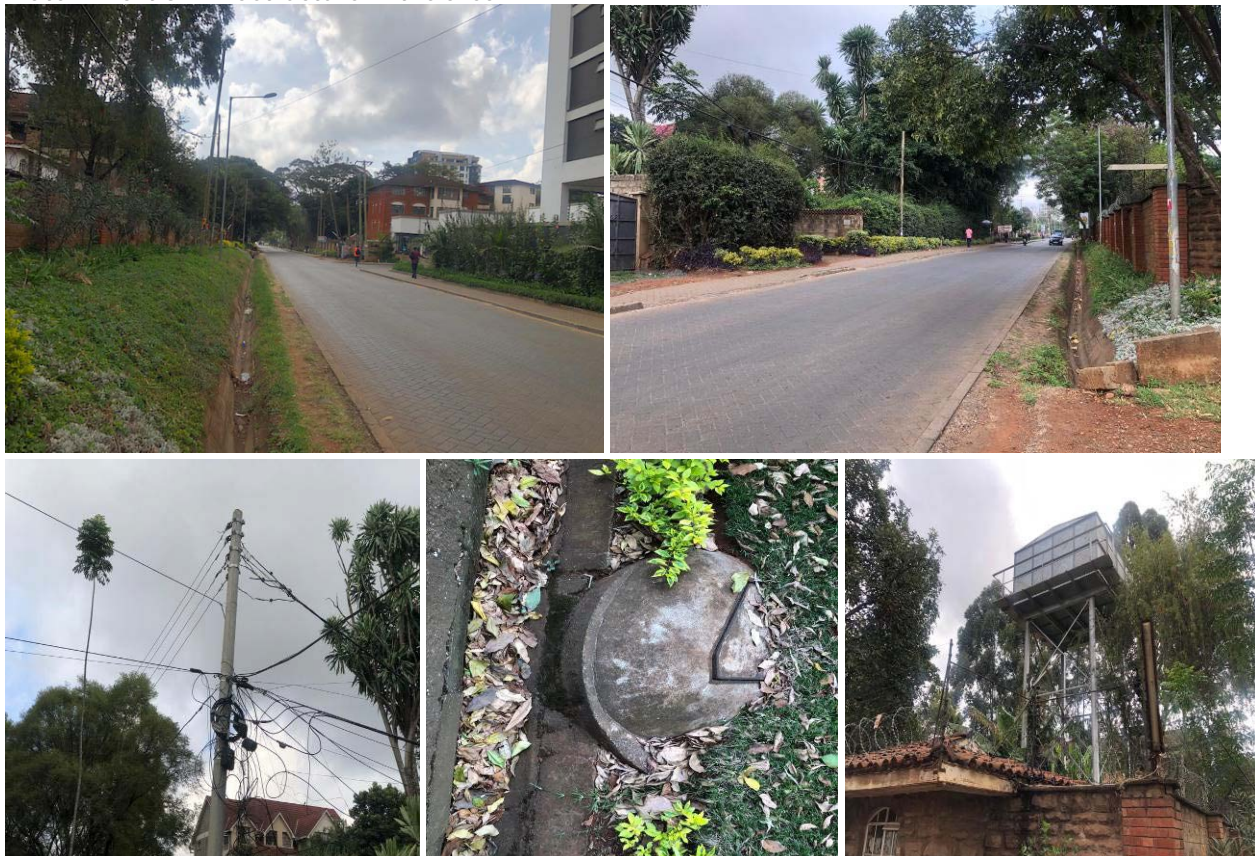
Plate 2: Part of infrastructure in the area
