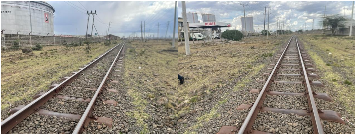
Photo 5 & 6: A section of the old railway lines serving the project site on both ends
