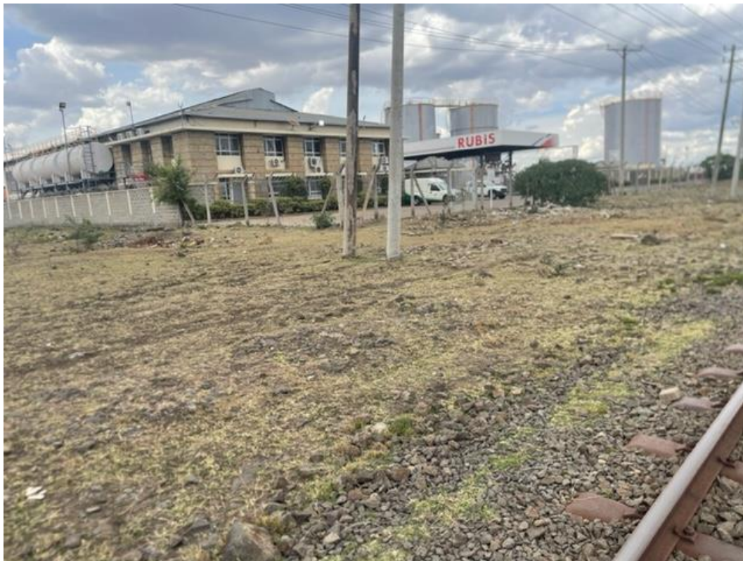
Photo 3: Rubis Energy Kenya Limited depot
