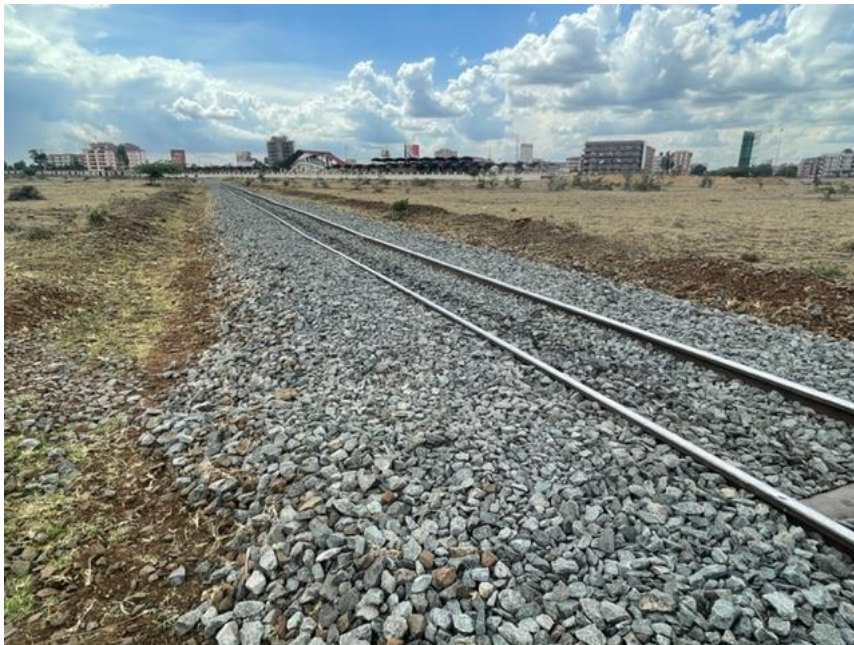
Photo 7: A section of the new railway lines serving the project site on South end
