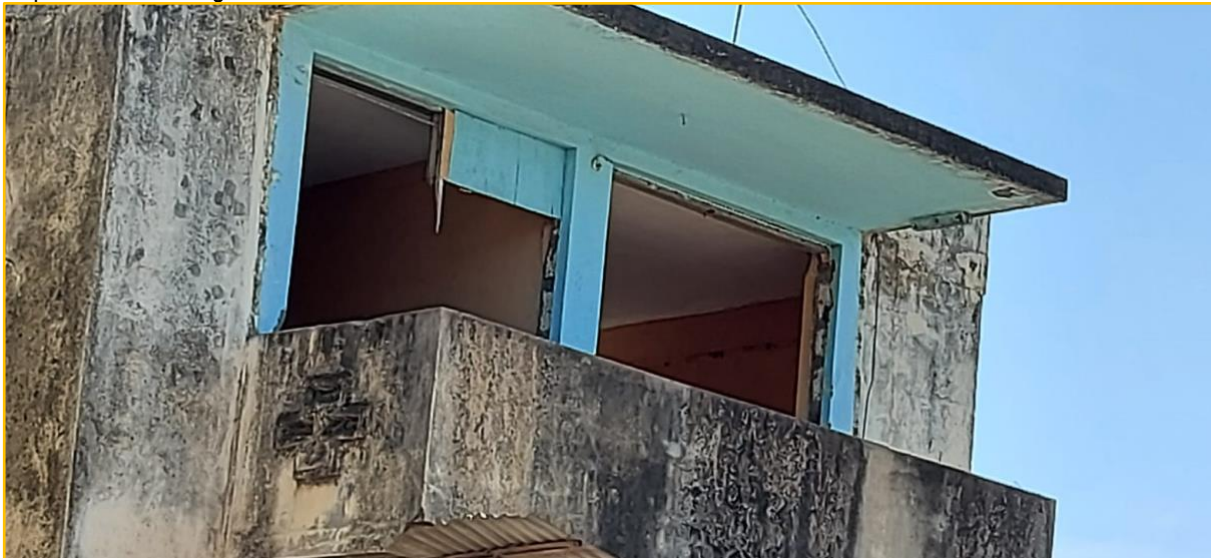
Plate 3 Recovery of doors & windows from Likoni flats housing units
