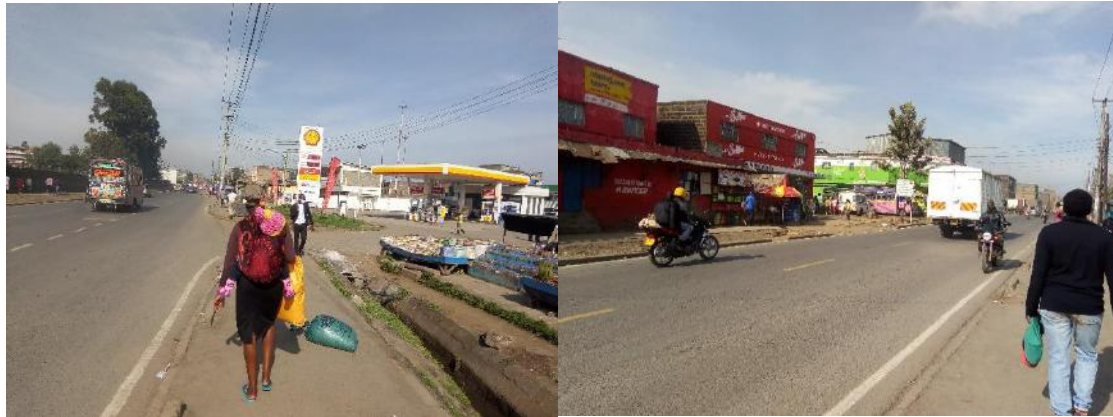
Picture 10 and Picture 11: Commercial structures at LR. 36/V/24 and at Lr No 36/I/261
