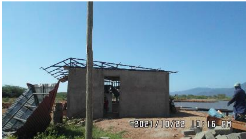
Figure 2-11: Powerhouse under construction
