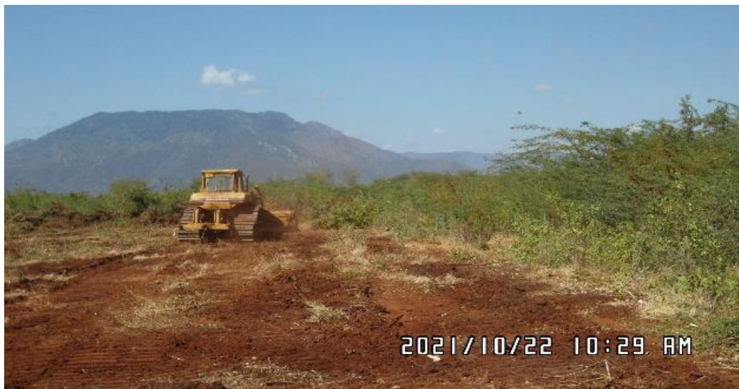
Figure 2-12 On-Going Clearing of Bush and Levelling of grounds
