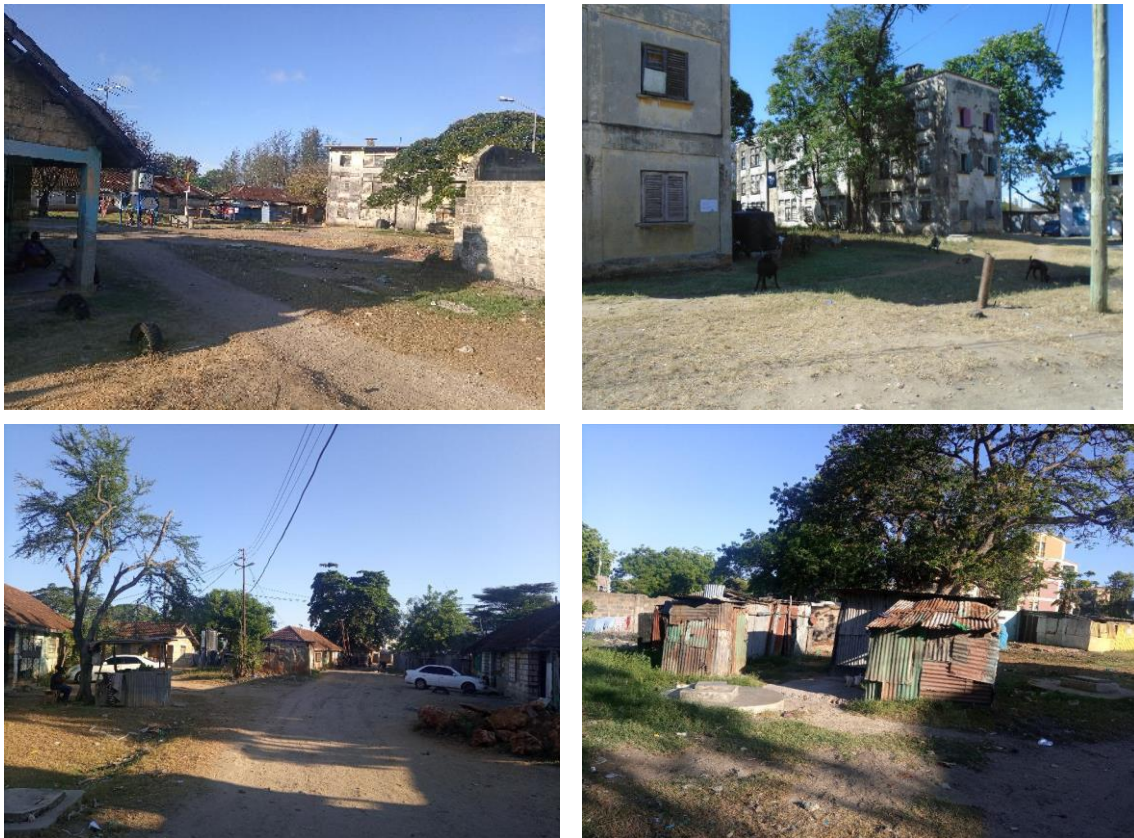
Plate 6: Existing houses and make shift structures at Mzizima Estate
