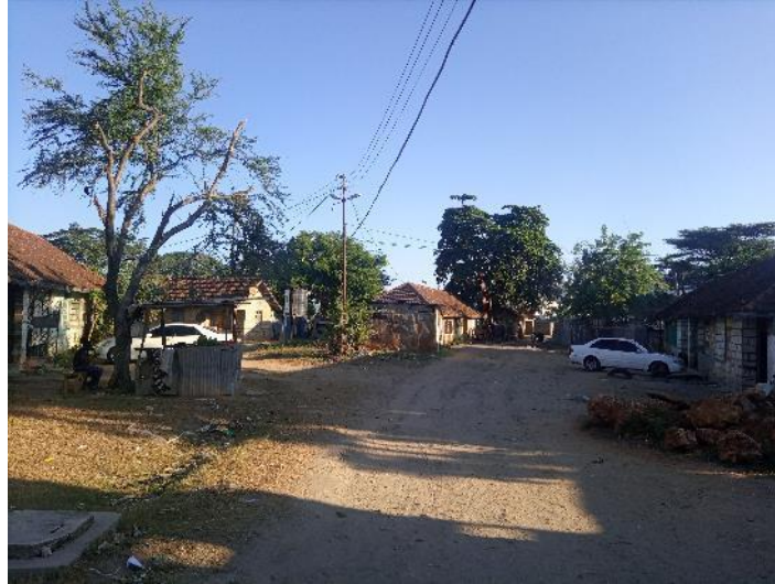
Plate 11: Power lines within the estate
