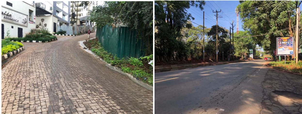
Plate 2: Part of infrastructure in the area
