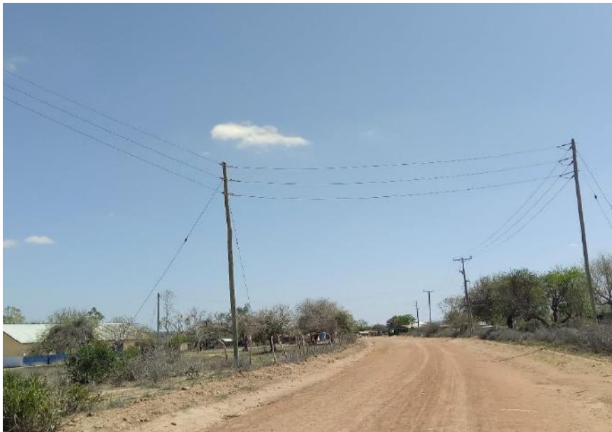
Figure 10: Electrical connectivity within the Makamini trading centre (Source: Field Survey, 2021)
