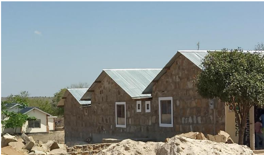
Figure 11: Permanent structure within Makamini trading centre (Source: Field Survey, 2021)
