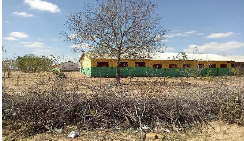
Figure 5: Makamini Primary School (Source: Field Survey, 2021)
