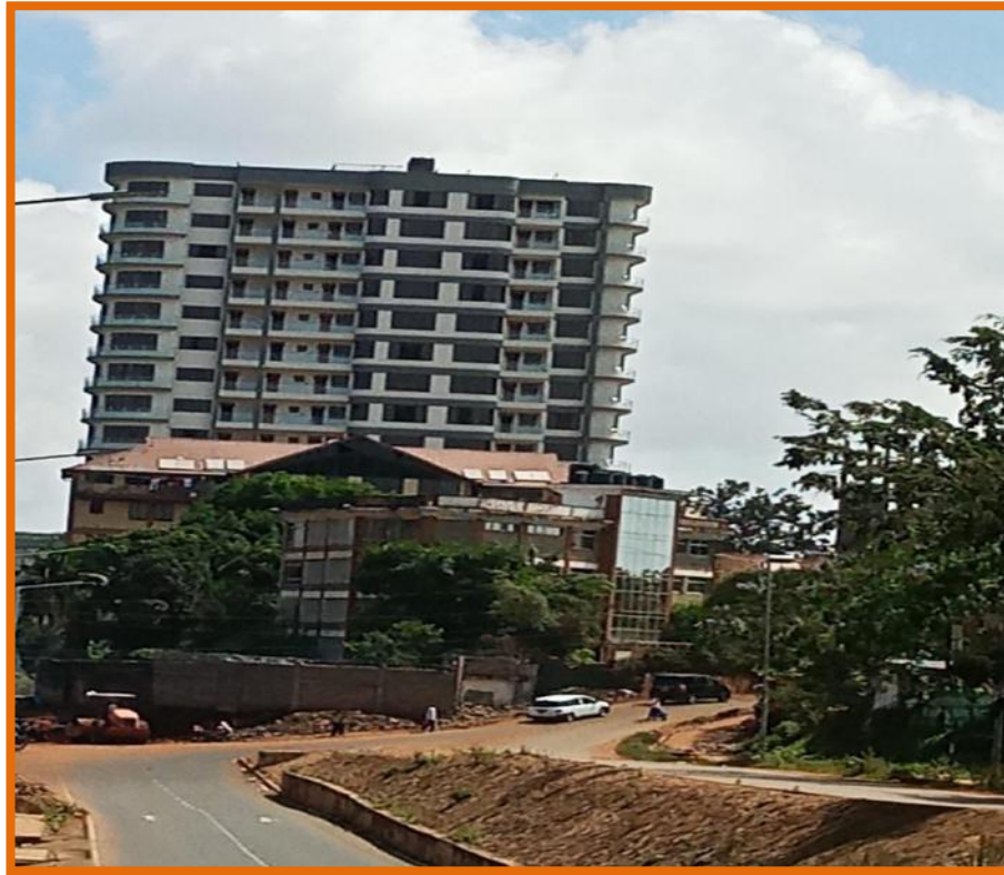
Picture 12: Other high-rise residential buildings in the neighbourhood.
