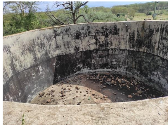
Plate 6-4: Concrete tank (0°24'28.54"S 36°15'25.05"E)
