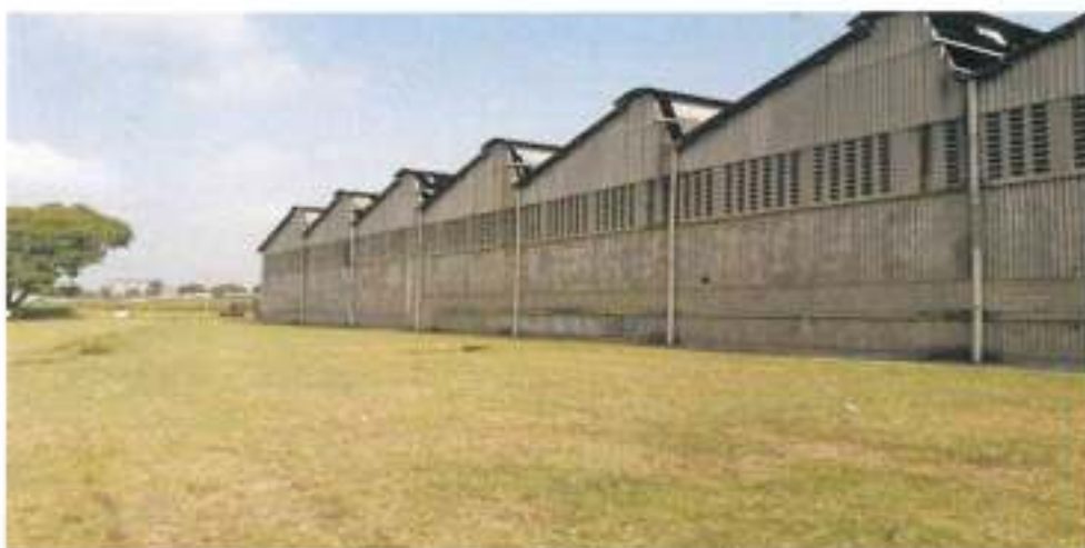
Figure 6: Loco shed with Asbestos roofing sheets at Nakuru Railway station
