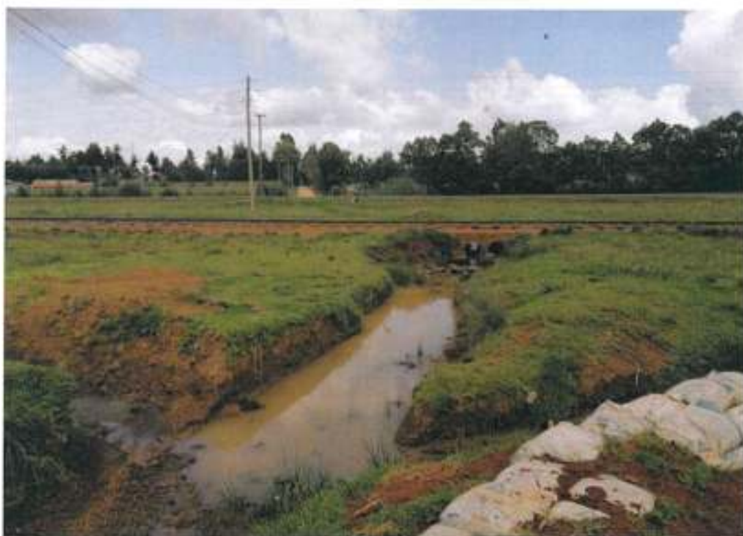
Figure 3: Clogged drainage culvert
