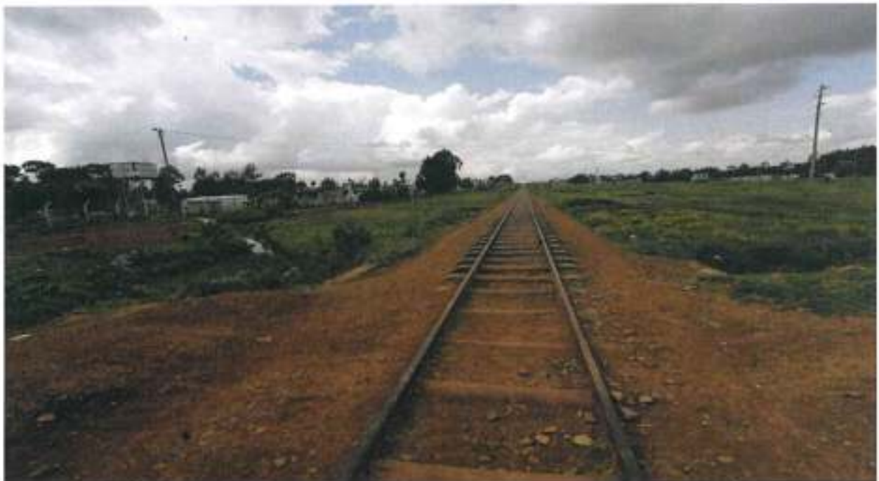
Figure 4: Silted rail track
