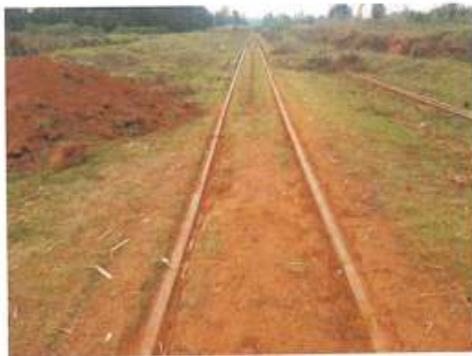
Figure 3: A section of the existing MGR line covered with soil at Bungoma- Malaba Section
