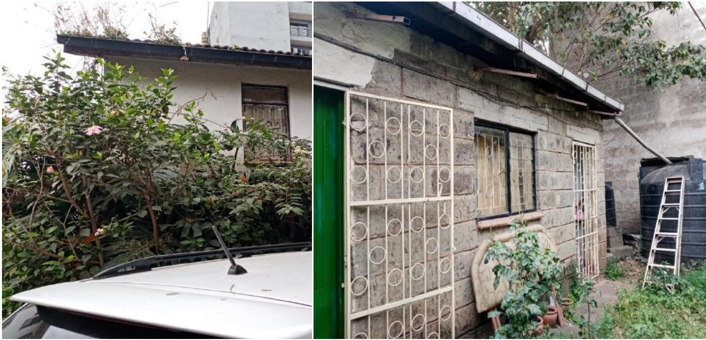
Figure 11: Existing Building Structures on Site
