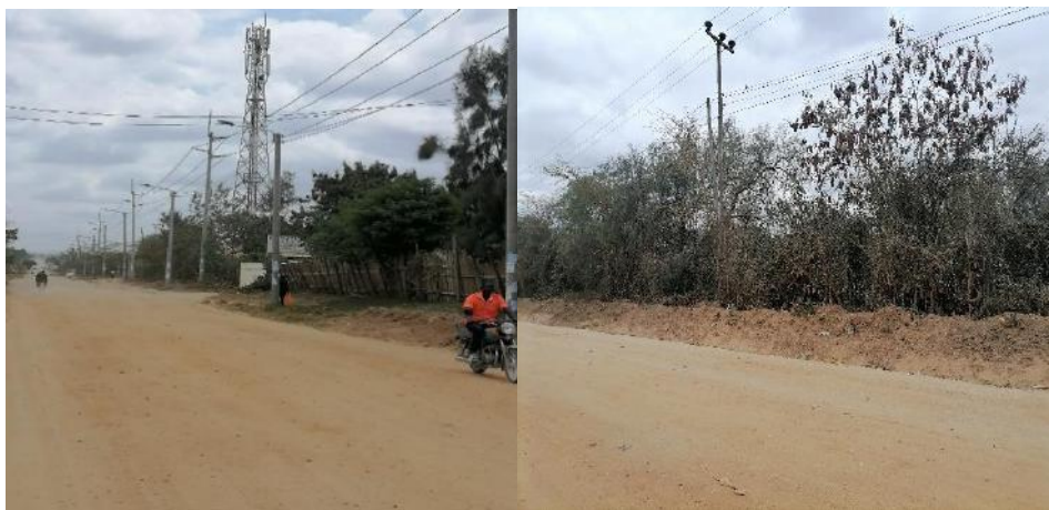
Figure 3-4 Old Namanga Road and electricity pole on the project site
