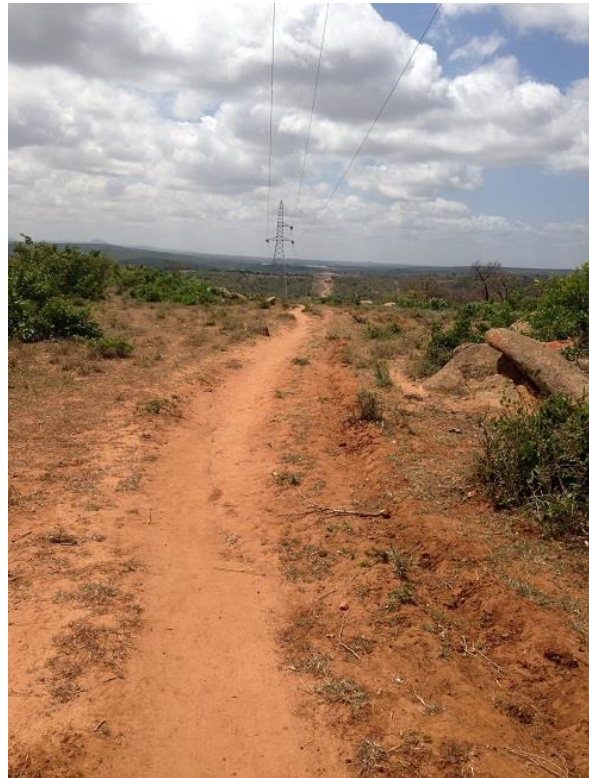
Plate 2.12: Section of an old TL way-leave corridor cleared of bushes; Courtesy of KETRACO
