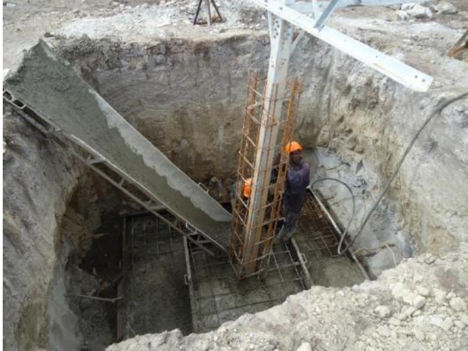
Plate 2.13: Tower foundation; Courtesy KETRACO
