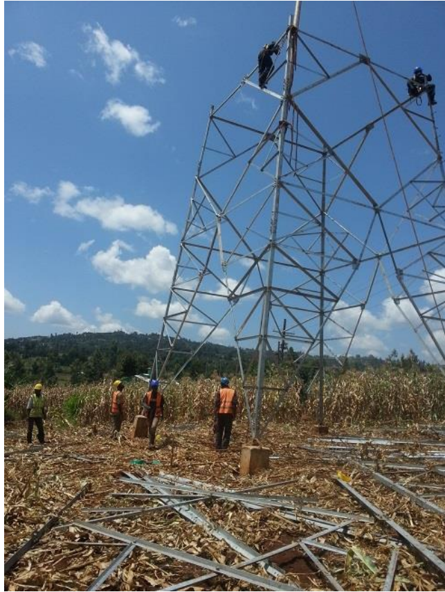
Plate 2.14: Tower erection; Courtesy of KETRACO
