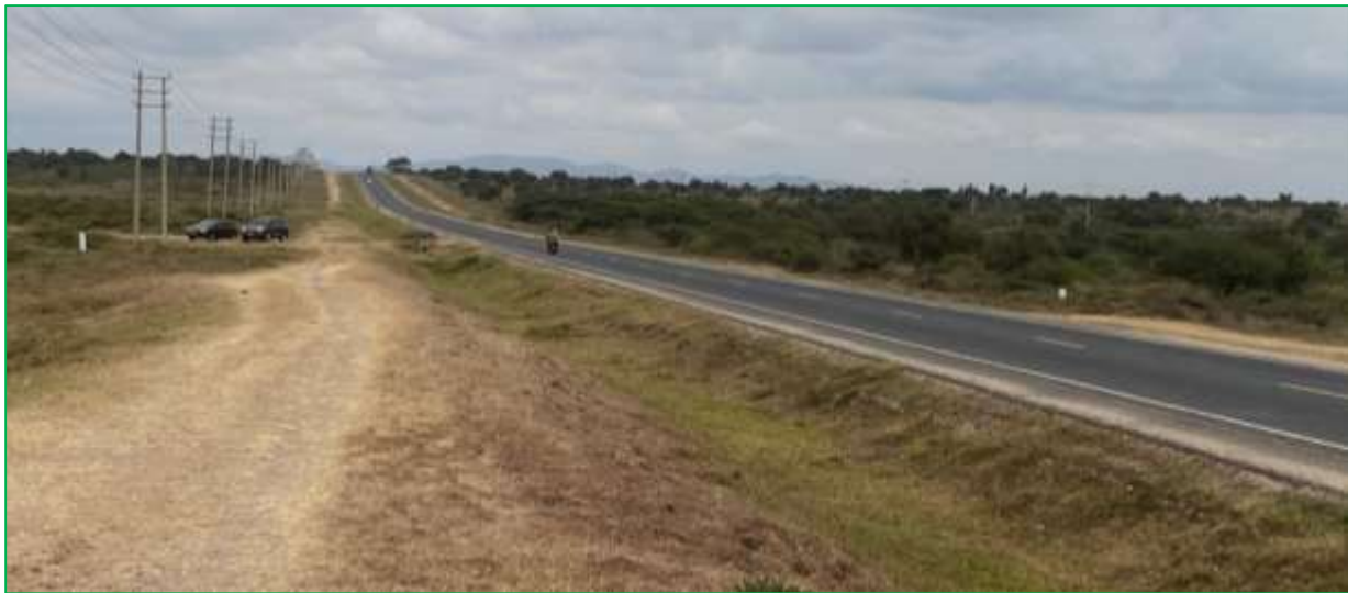
Figure 12: A section of Nairobi – Namanga Highway (Source: Site visit, July 2021).
