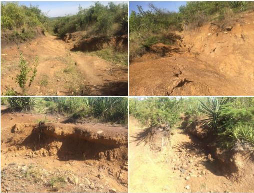
Plate 35 Gulley erosion at the Gogo hydropower expansion project site
