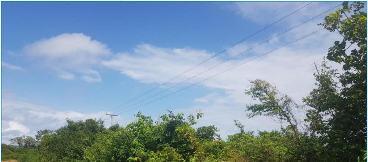
Figure 18: Power supply lines near the proposed project site (Source: Site visit, July 2021).
