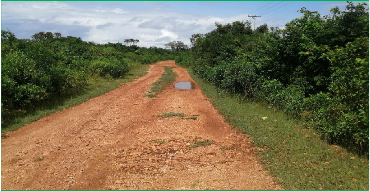
Figure 17: A section of the access earth road; Fikirini- Kibuyuni road (Source: Site visit, July 2021).
