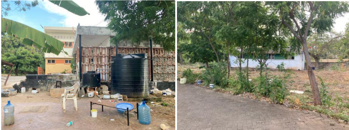
Plate 3 Existing buildings on the project site.
