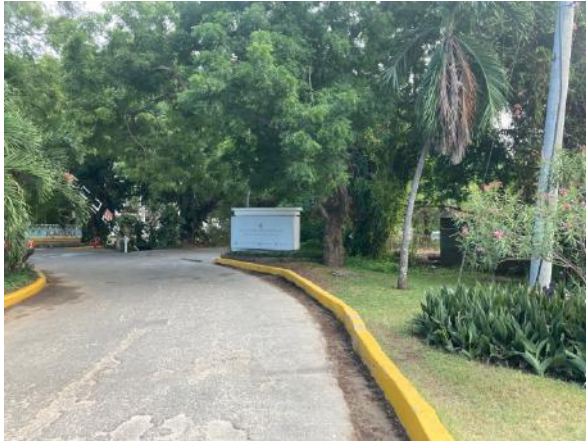
Plate 6 Project site all-weather access road
