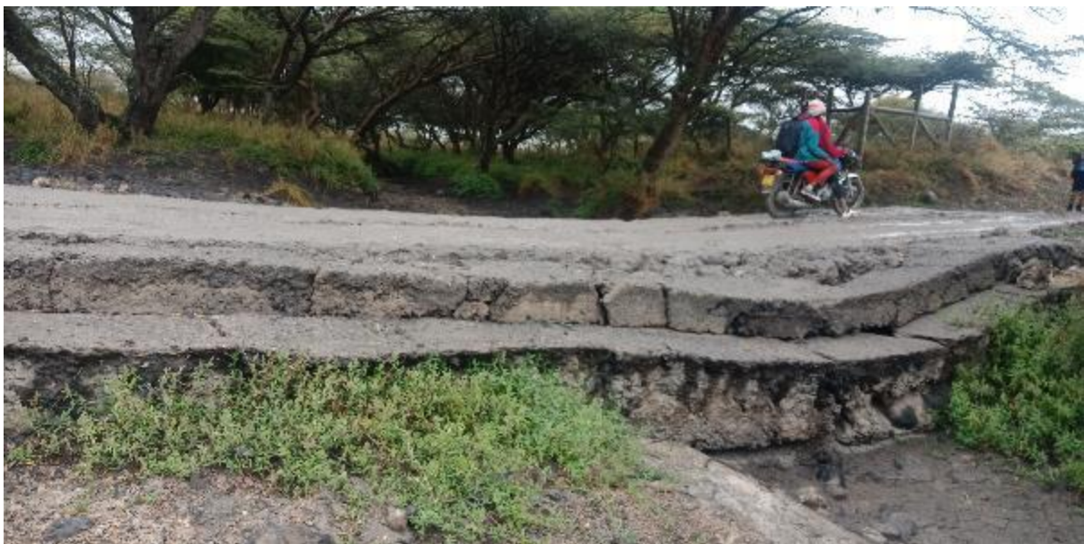
Plate 17: Constructed drifts along the proposed road project which get affected during heavy rains
