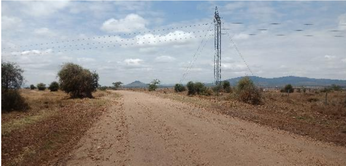
Plate 9: High powered cables crossing the project road at Malili town
