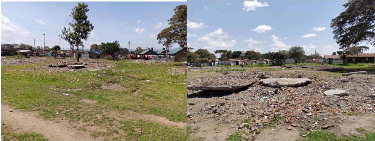
Partly demolished parts of dilapidated government housing
