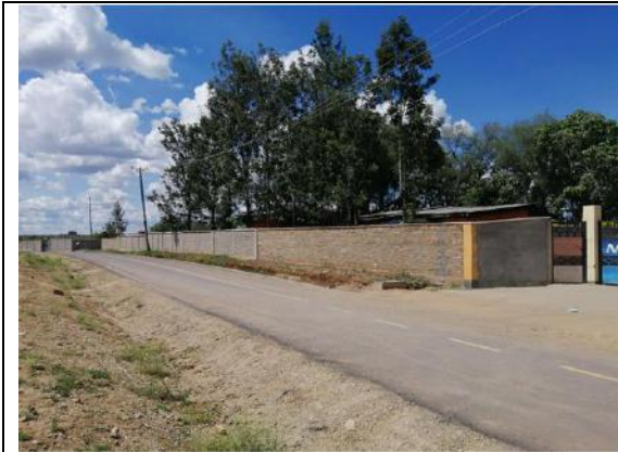
All-weather access road/perimeter wall for Moke Gardens
