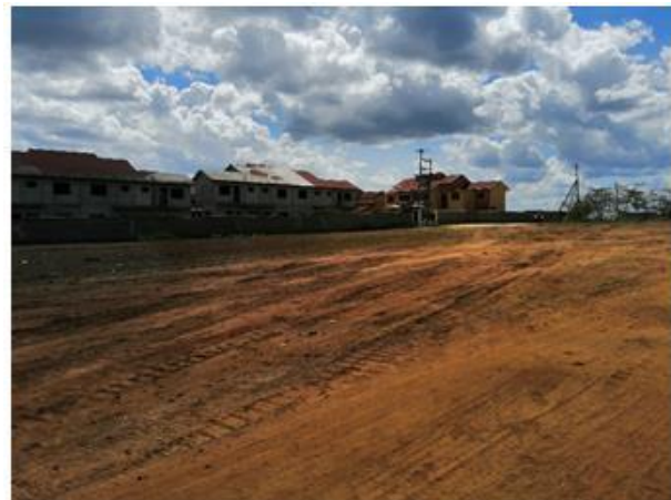
Existing maisonettes adjacent to the project site
