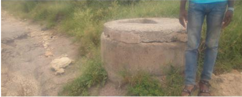
Figure 4-7: Conventional Sewer Manhole along the 18m Road
