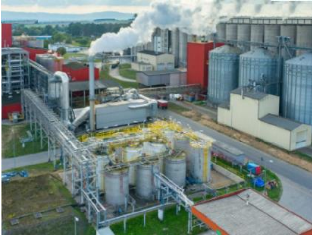
Figure 34: Typical Emission - Bamburi cement Image source ( https://www.afrik21.africa/ )
