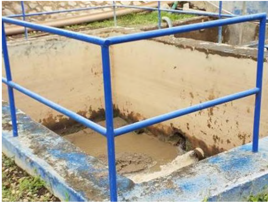
Figure 6.3: Sludge collected in sludge chambers at the site
