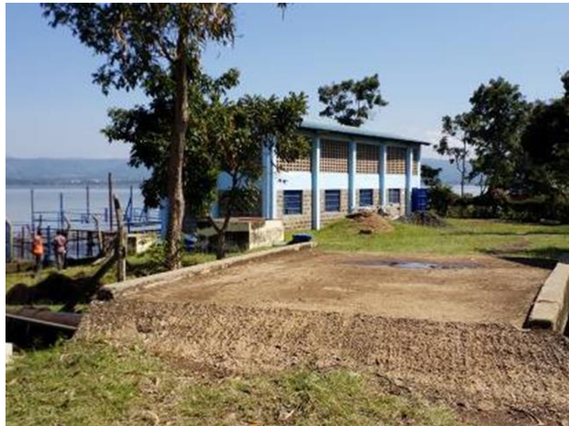
Figure 3.1 2007 and 2011 pumping station
