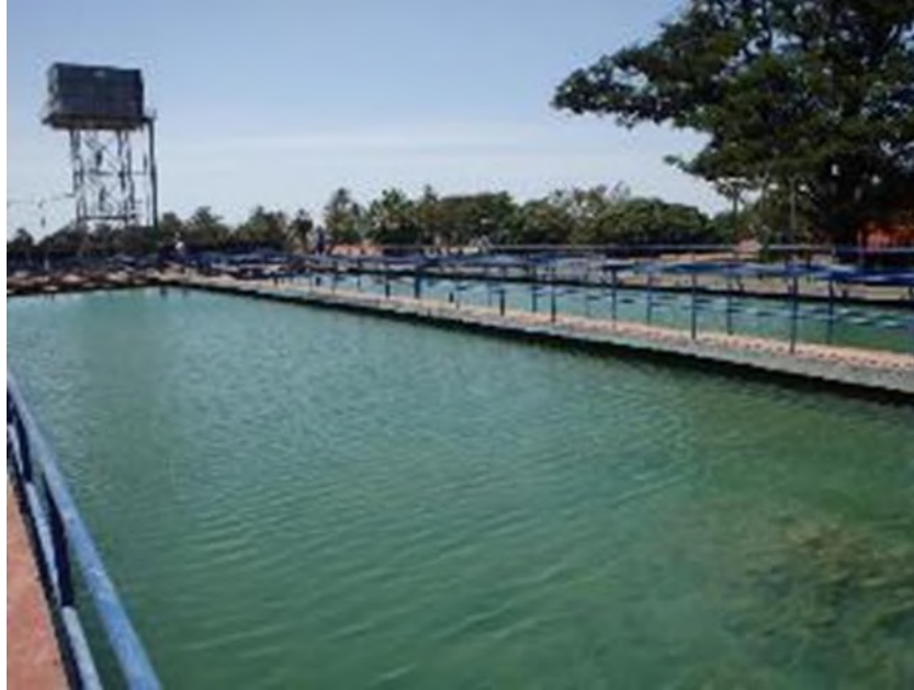
Figure 3.3: Sedimentation basin (new line)
