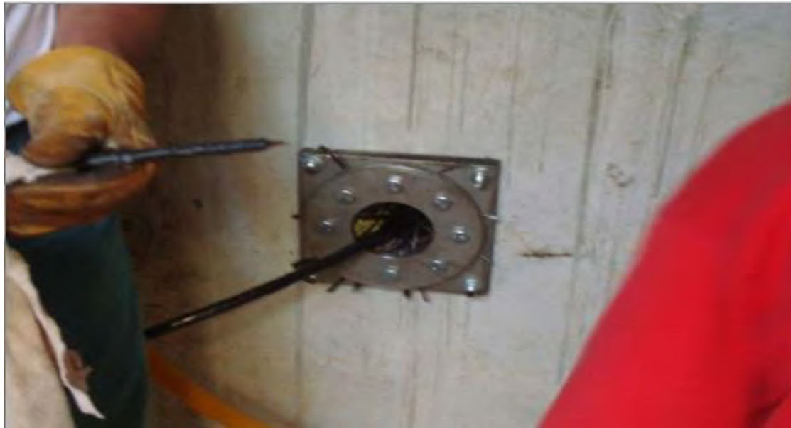
Photo 2-7 Applying permanent manhole stopper
