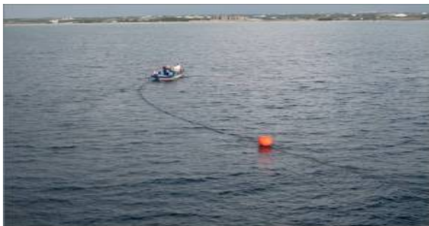
Photo 2-2 Messenger rope hauling to the beach
