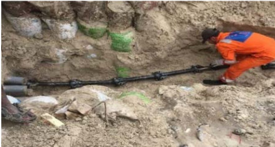
Photo 2-8 Articulated pipes installation
