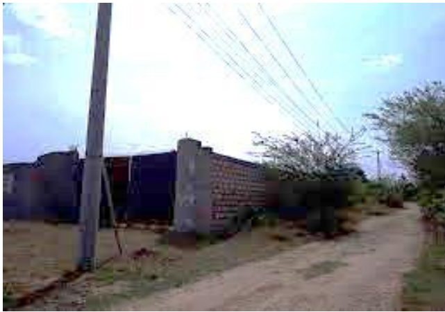
INSET: A Three Phase Power Line Accessible Near The Site Installed By KPLC.
