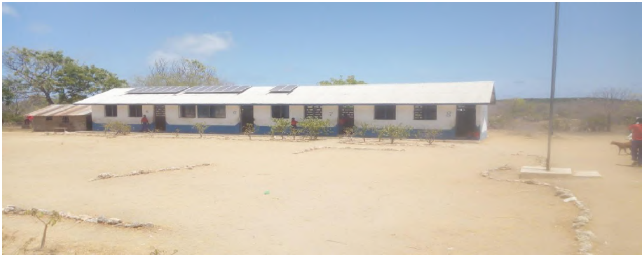
Figure 23: Use of solar energy in Kiongwe village
