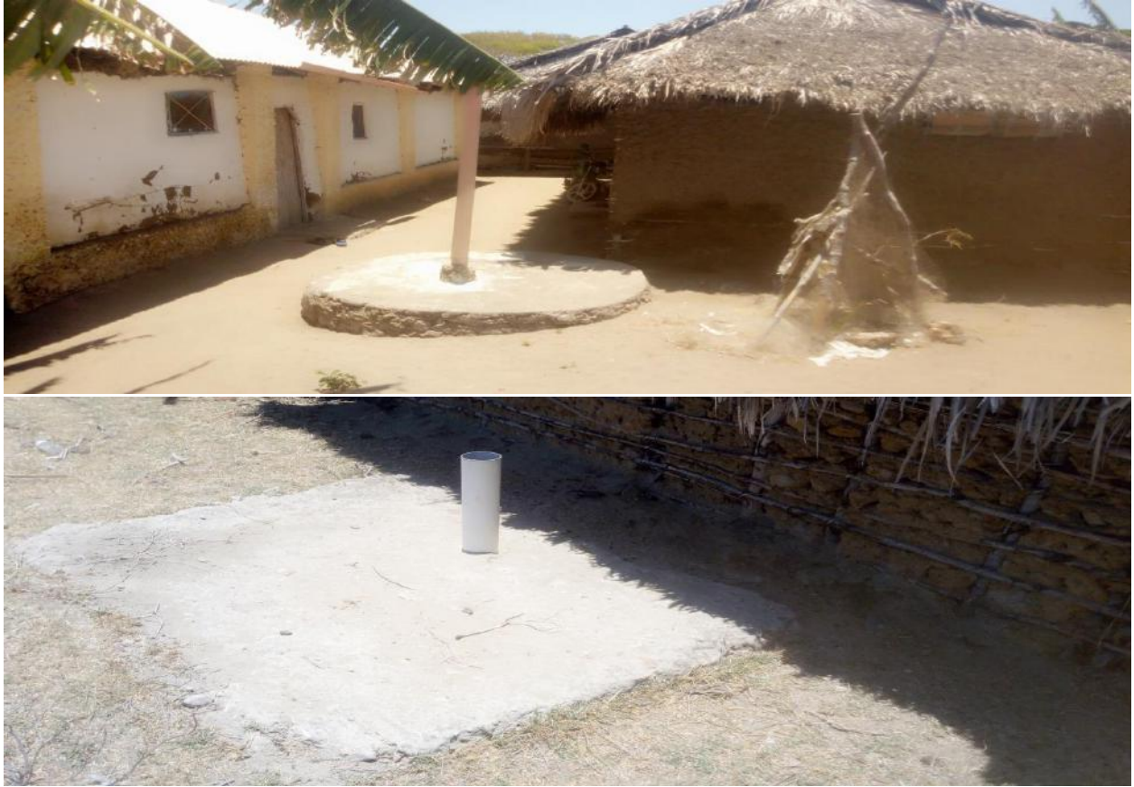
Figure 33: Septic tanks used to manage liquid human waste at Kiongwe village
