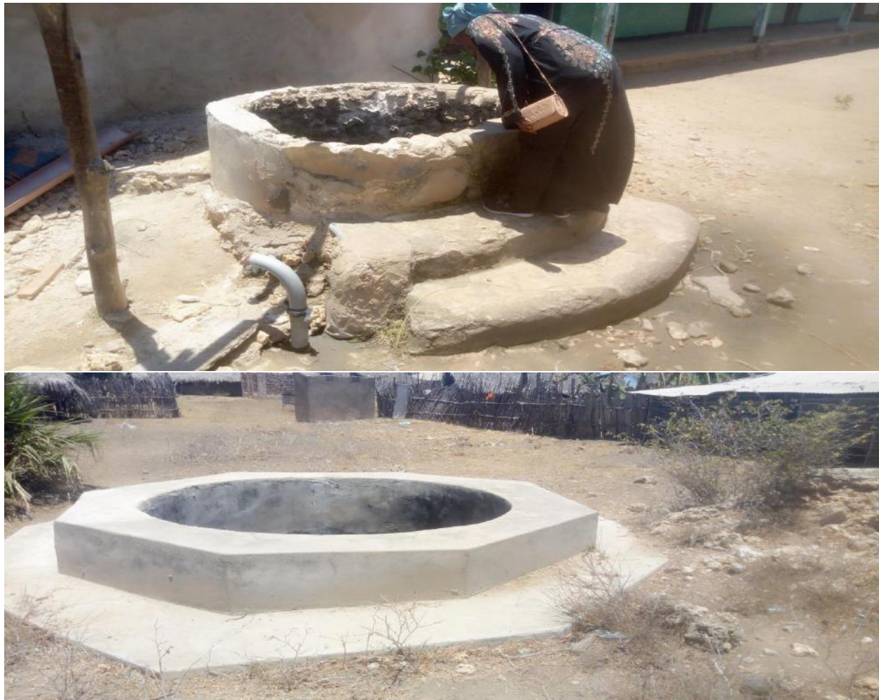
Figure 31: Water wells at kiongwe village
